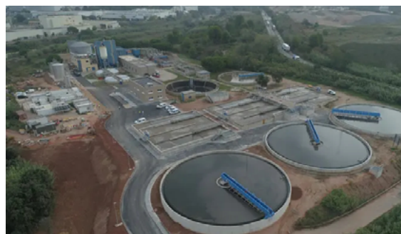
Rubí wastewater treatment plant.
